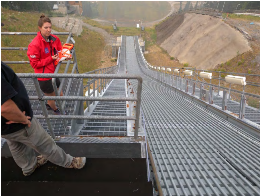
protruding fence at end of entrance stairs – cover with soft mat
