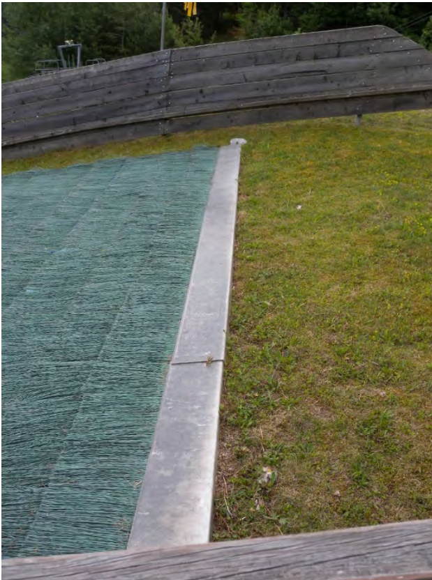
hard fixing edges at beginning of mat covering
