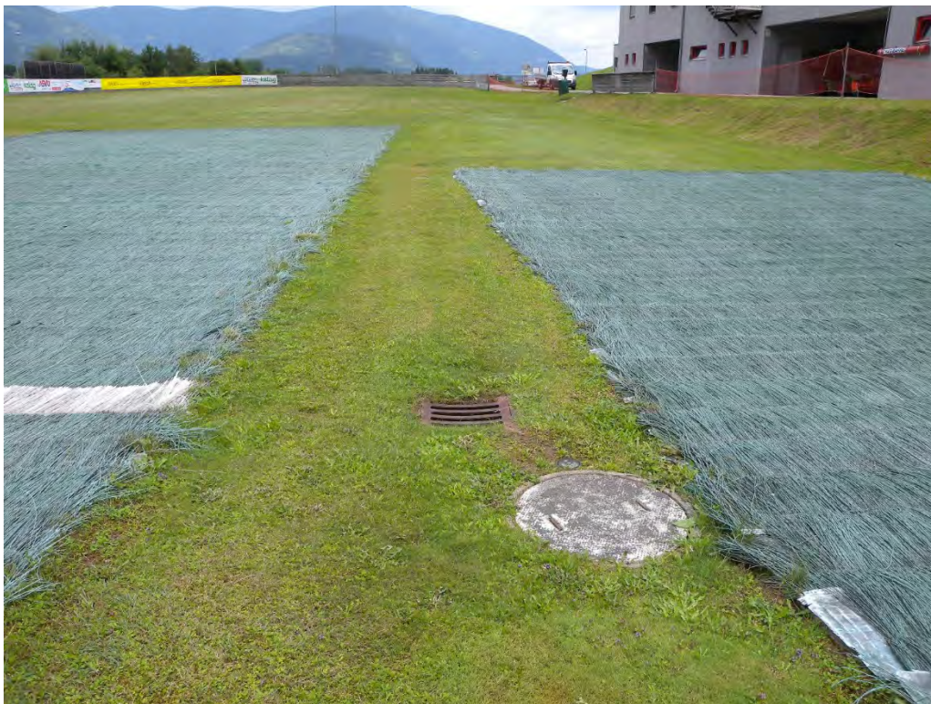
dewatering shafts with slots in outrun
