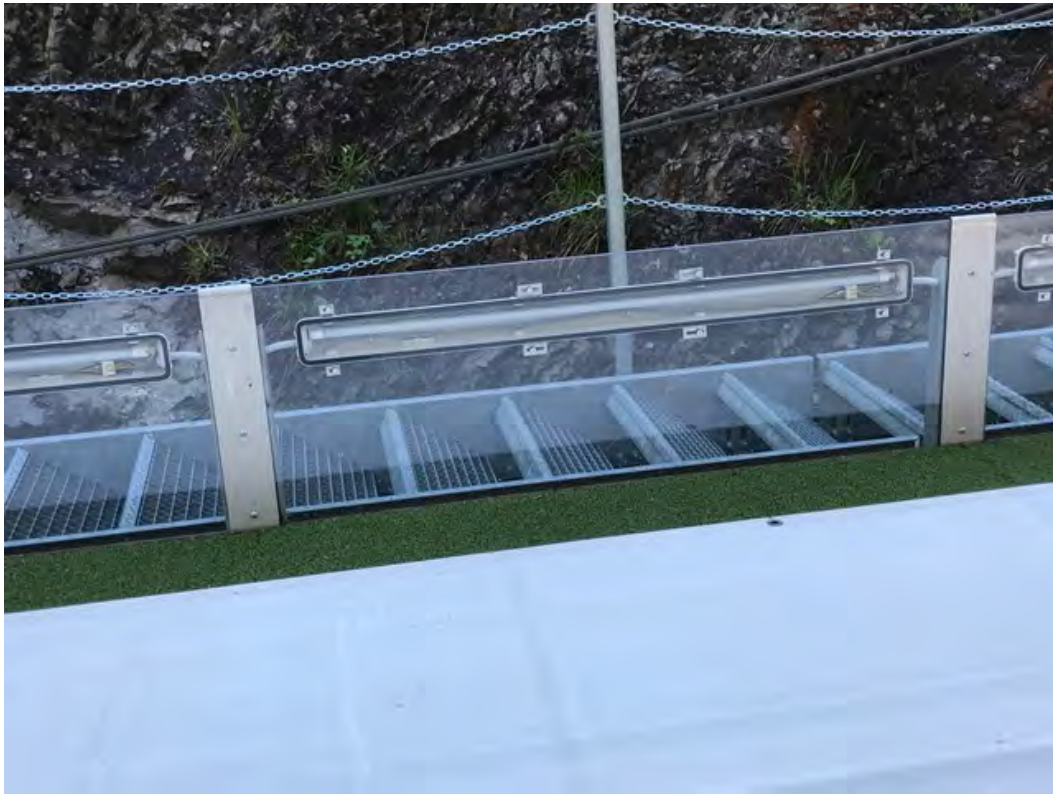
lamps mounted outside of plexiglass sideboards – shining through glass – OK
