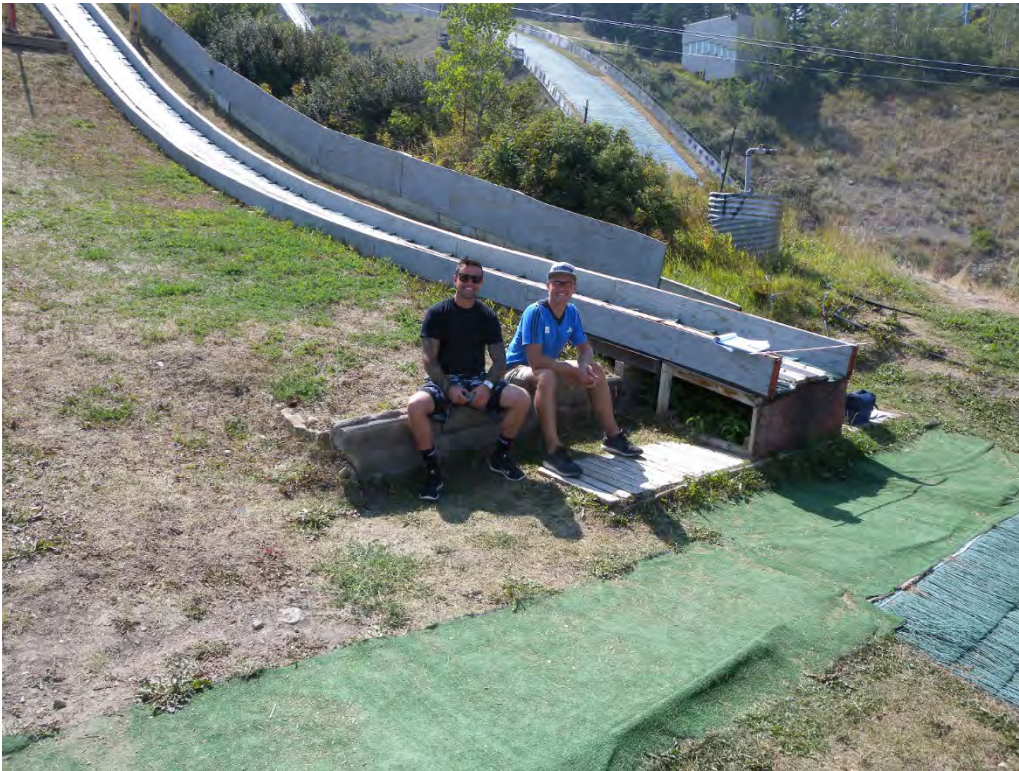
free space for fallen athlete besides inrun, but protect concrete blocks with a (soft) fence to prevent bumping down of athlete and to catch loosened skis
