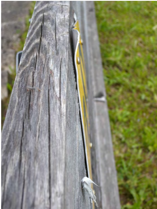
metering numbers with sharp edges
