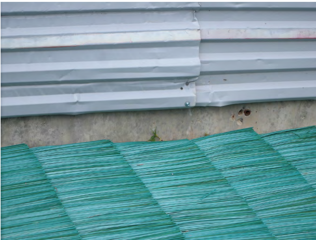
concrete basement to be covered
