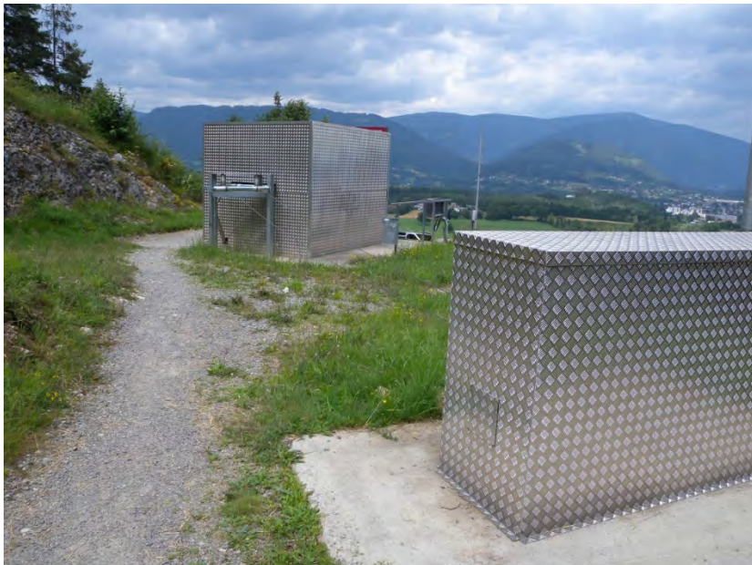
if steel rope brakes, pedestrians on footpath are highly endangered
