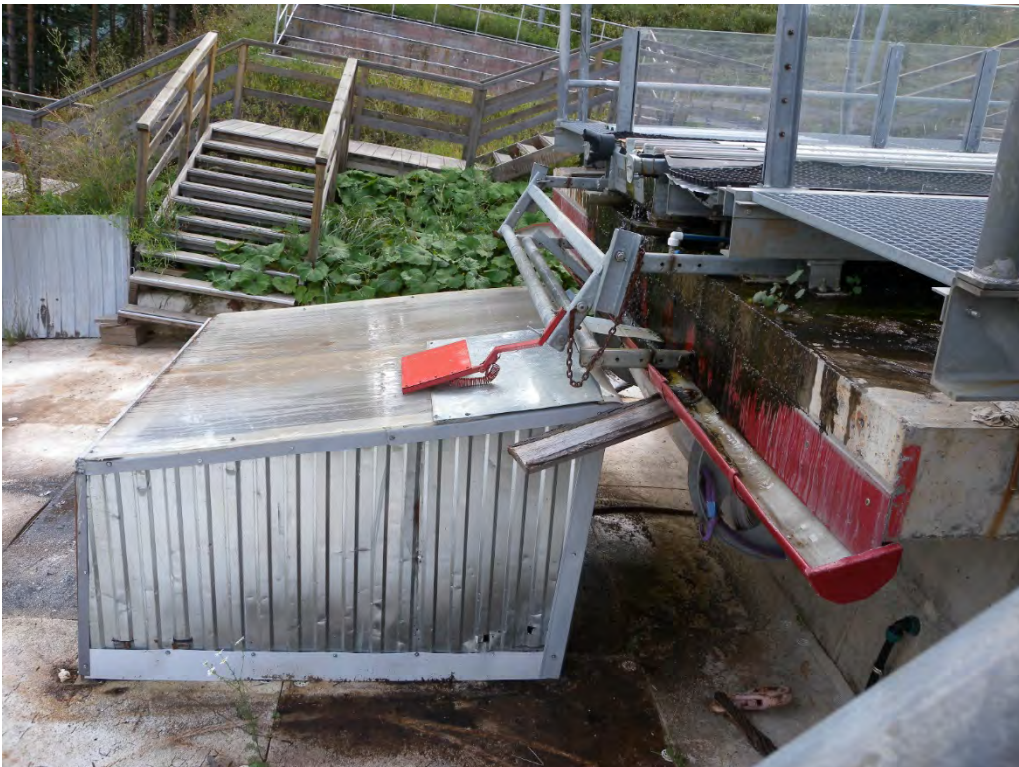
storage building underneath the table
