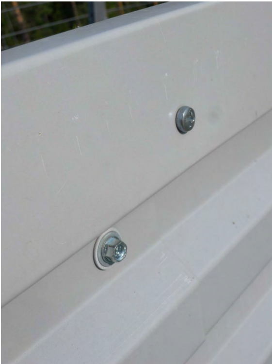
protruding screw heads
