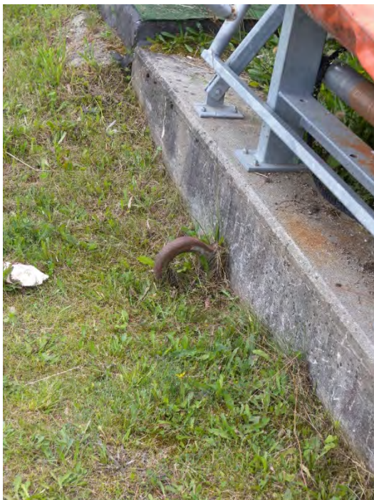
during summertime cover steel fixing eye for preparation machine
