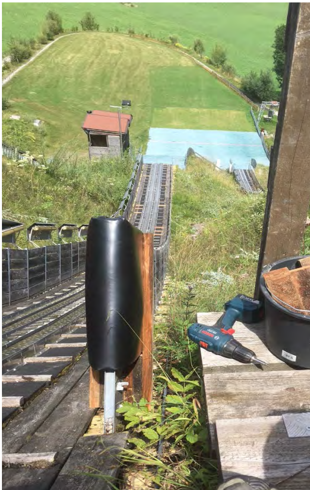
protruding wooden latches besides inrun track, soft mat too short
