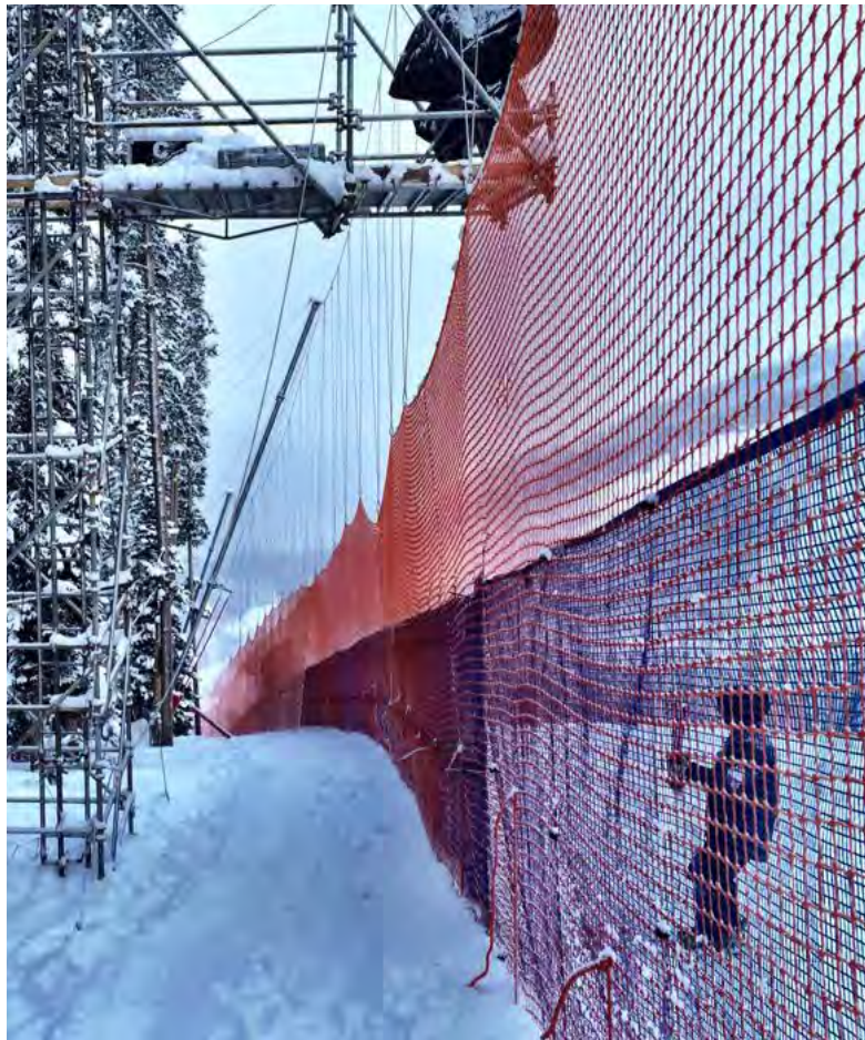
scaffolding fitting with permanent A fences
